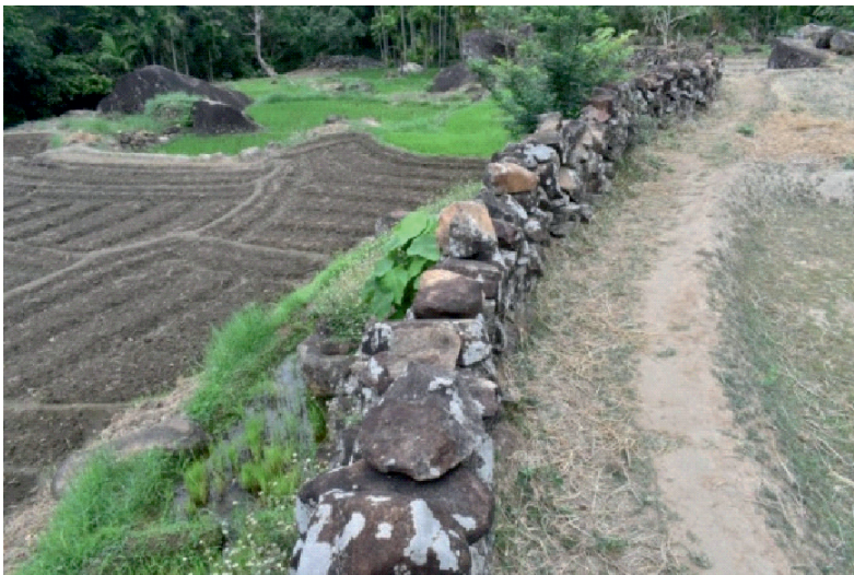
Photo 08: Rear view of the stone wall and gate separating Gamwela and Uda paddy field
