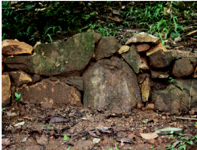
Photo 01: Erosion barrier
