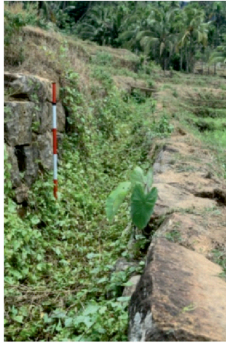
Photo 10: Canal falling through the middle of the paddy field
